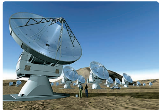
FIGURE 1 Artist's rendition of the ALMA radiotelescope, which will consist of up to 64 12-meter parabolic antennas spread over 18 km. The array will receive cosmic signals from 31–950 GHz. Image courtesy of NRAO/AUI and computer graphics by ESO.
